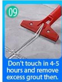
09 Don't touch in 4-5 hours and remove excess grout then.
